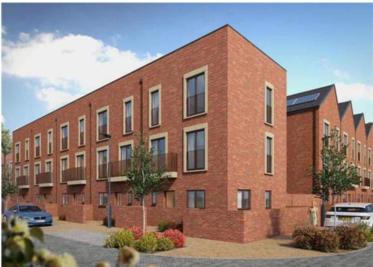
Electric Quarter Phase 1 completed in 2021
